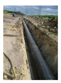
Direct backfill of the screened out finesize into the shaft of utility line
