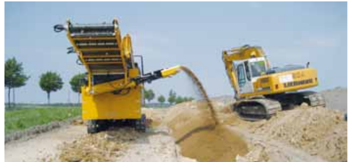
Use in pipeline construction with direct filling of the fine grain
